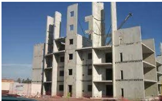
Figure 3. Illustrative photos of creating a prefabricated building
