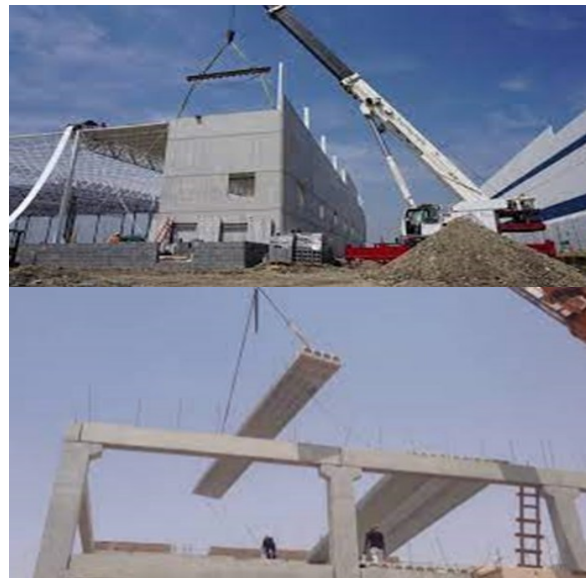
Figure 4. Illustrative photos of creating a prefabricated building
