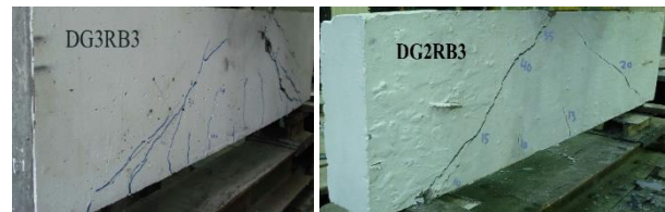
Figure 10: Crack pattern for directly loaded beams
