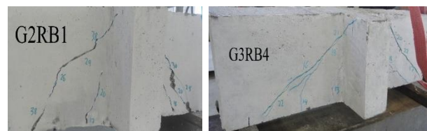
Figure 9: Crack pattern for indirectly loaded beams
