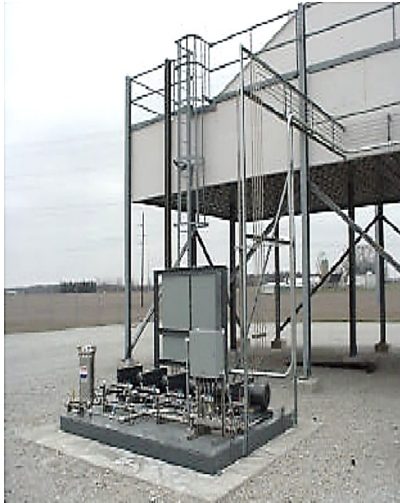
Figure 1. Typical fogging skid with high pressure. Here are the feed lines from the high-pressure pumps to the intake system [39]
