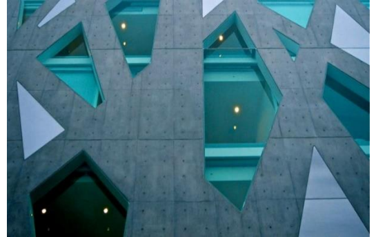
Fig (5) appearance of concrete material at elevation level [15]
