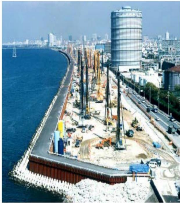
Figure 13. Application of DJM and resulting columns at Yodogawa River embankment in Japan(18)
