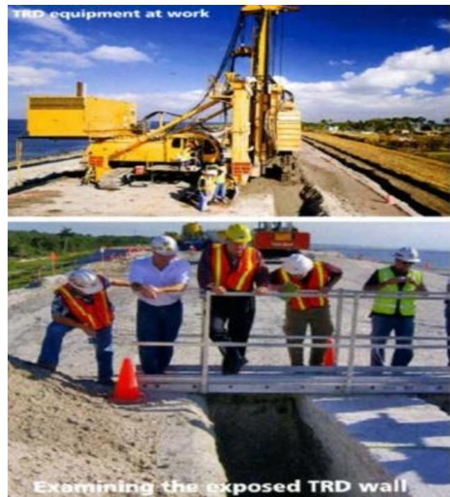
Figure 9. Top: TRD machinery in operation; Bottom: TRD wall inspection at Herbert Hoover Dike, which encircles Lake Okeechobee in southeast Florida[18]
