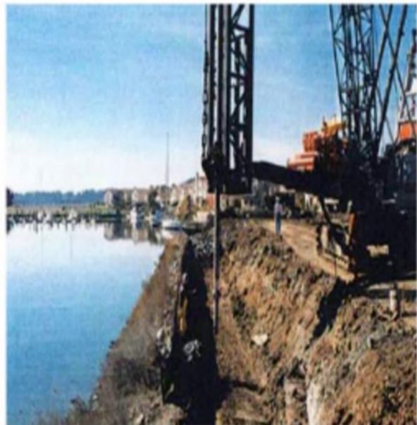
Figure 12. Liquefaction mitigation along river bank at Napa Yatch club, California[18]
