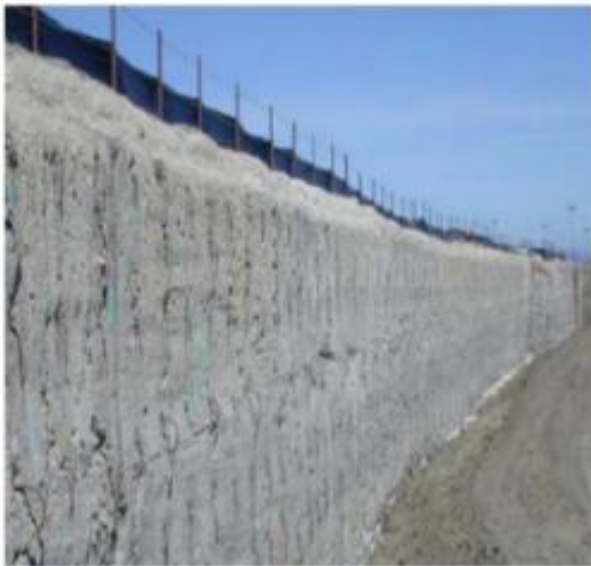
Figure 10. Reinforced deep mixing retaining wall[18]
