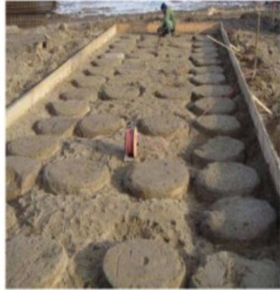
Figure 8. Foundation for Motorway Bridge near Katowice[18]
