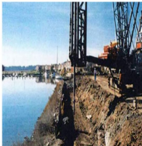
Figure 12. Liquefaction mitigation along river bank at Napa Yatch club, California[18]
