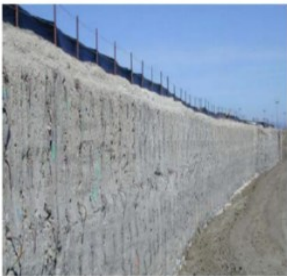
Figure 10. Reinforced deep mixing retaining wall[18]
